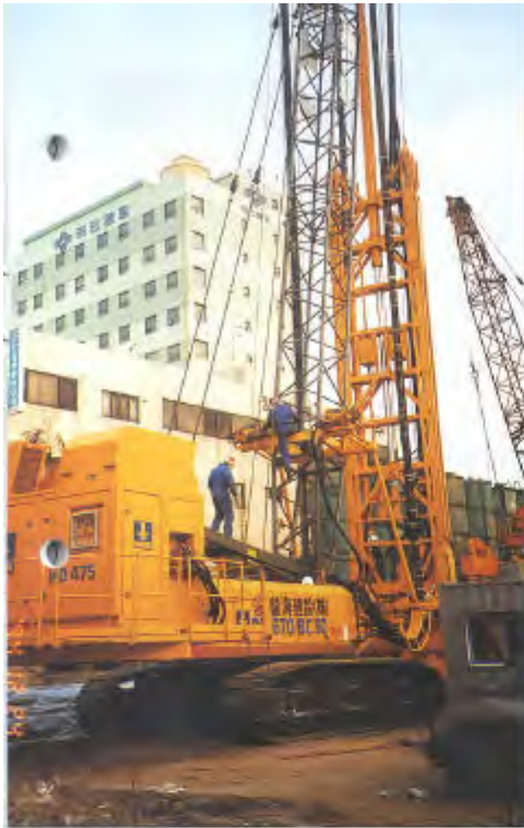
BC 30 on 80 hp - base machine, cutting depth 45 m
