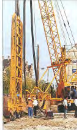
Rotation device on upper carrier (excavator). Rotation device on mast head (tower).
