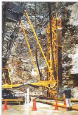
Rock Cutter on Shinkawa Dam in Japan
