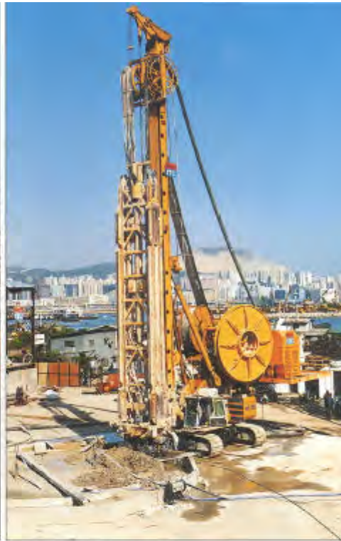
BC 30 on 110 hp BG 40, cutting depth 50 m
